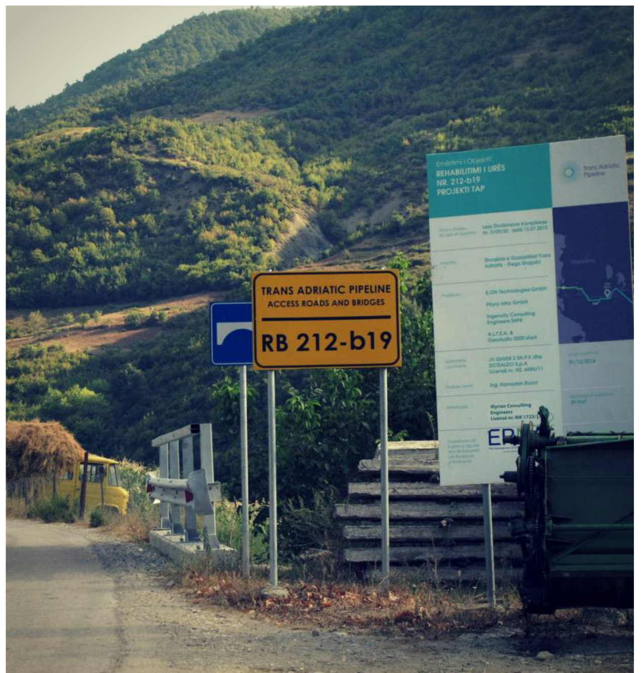
Roadside signs heralding TAP construction works. Buzuq, Albania. CEE Bankwatch Network
